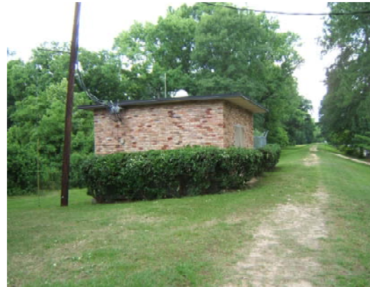
Storm water Pump Station atop the river levee
