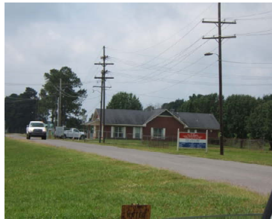
Wastewater Treatment Plant on Richwood Rd. #2
