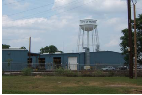
The Water Treatment Plant on Grammont Street
